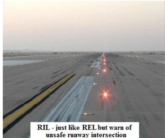
Figure 6: Runway Intersection Lights
